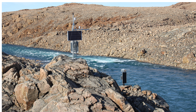
Figure 4. Automated weather station and CF bubbler with a vented pressure transducer (on the left) and a time-lapse camera (on the right) established at the Minturn River. Other instruments at this site include two bank-mounted laser rangefinders, a second vented pressure transducer, and a second time-lapse camera on the opposite bank (photo credit: Lincoln Pitcher).
