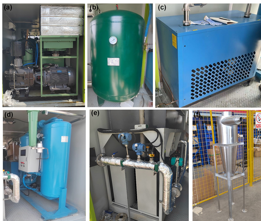
Figure 3. Main components of the air system: (a) air compressor; (b) air receiver; (c) freezing dryer; (d) desiccant dryer; (e) air cooler, 1-flowmeter, 2-dew-point hygrometer, 3-manometer, 4-temperature sensor; and (f) cyclone dust collector.
