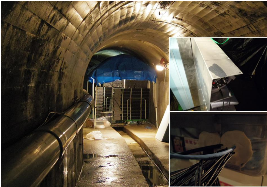
Fig. 5. Photograph of the muon radiography measurement system in the drain tunnel and a housing of the muon readout module (bottom inset). The top inset shows dew condensation on the scintillation counter bar.
