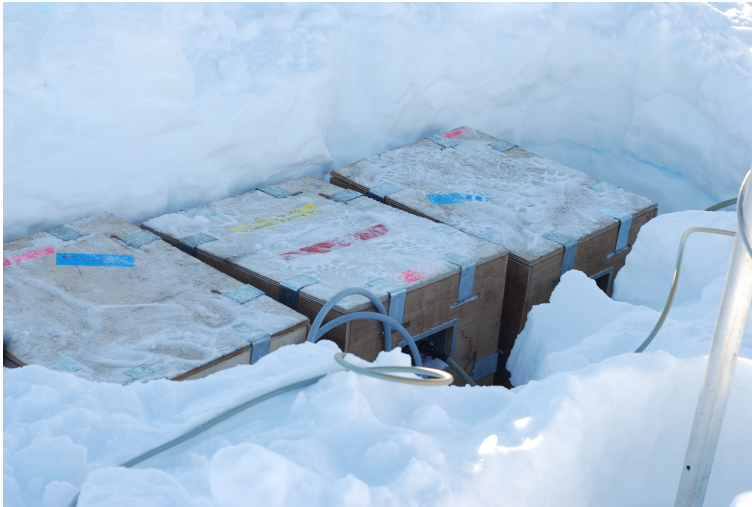
Figure 2. 6 100 Ah batteries in 3 battery enclosures, for the field installation of Fig. 1. In total, the batteries and enclosures weighed 300 kg, nearly half of the aircraft payload available for the site installation.
