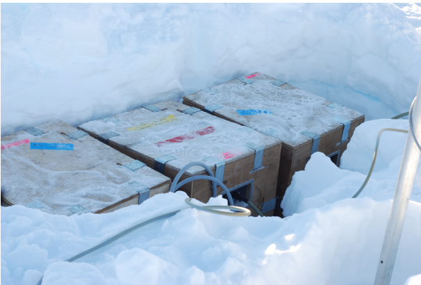
Fig. 2. 6 100Ah batteries in 3 battery enclosures, for the field installation of figure 1. In total, the batteries and enclosures weighed 300kg, nearly half of the aircraft payload available for the site installation.
