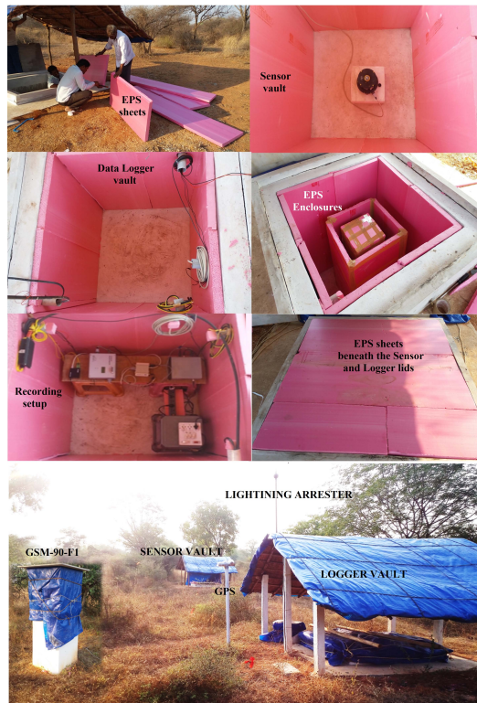
Fig. 2. Figure 02. Thermally insulated new variometer vaults using Extruded Polystyrene (EPS) foam sheets for good temperature control and the location of sensor and logger vaults.
