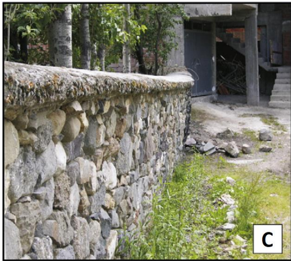
Figure 6. Aseismic creep sites (a)at Ismetpasa railway station, and (b) damaged brick-wall at Hamamlı village close to Ismetpasa. (c) Out-bended wall at Destek village (from Karabacak et al. 2011).
