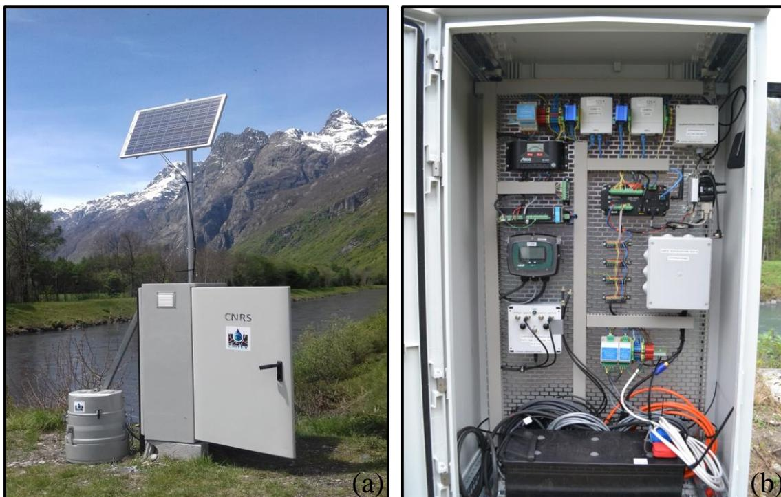
**Figure 3 : Photos of the box that houses all the electronics of the platform and the battery: (a) outside view where we also see the solar panel and the ISCO automatic river water sampler, (b) inside view.**
