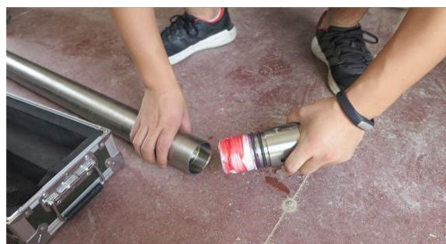
Figure 23: Seal and install the threaded joint.
