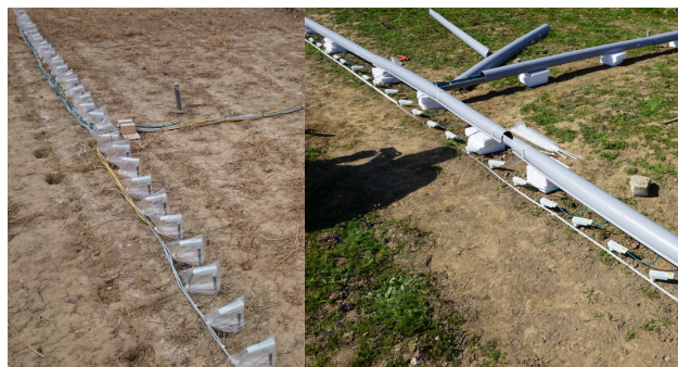
Figure 4. Installation of electrodes, electrode modules, and connecting cables. Left: Installation in 2017, right: Installation in 2018.
