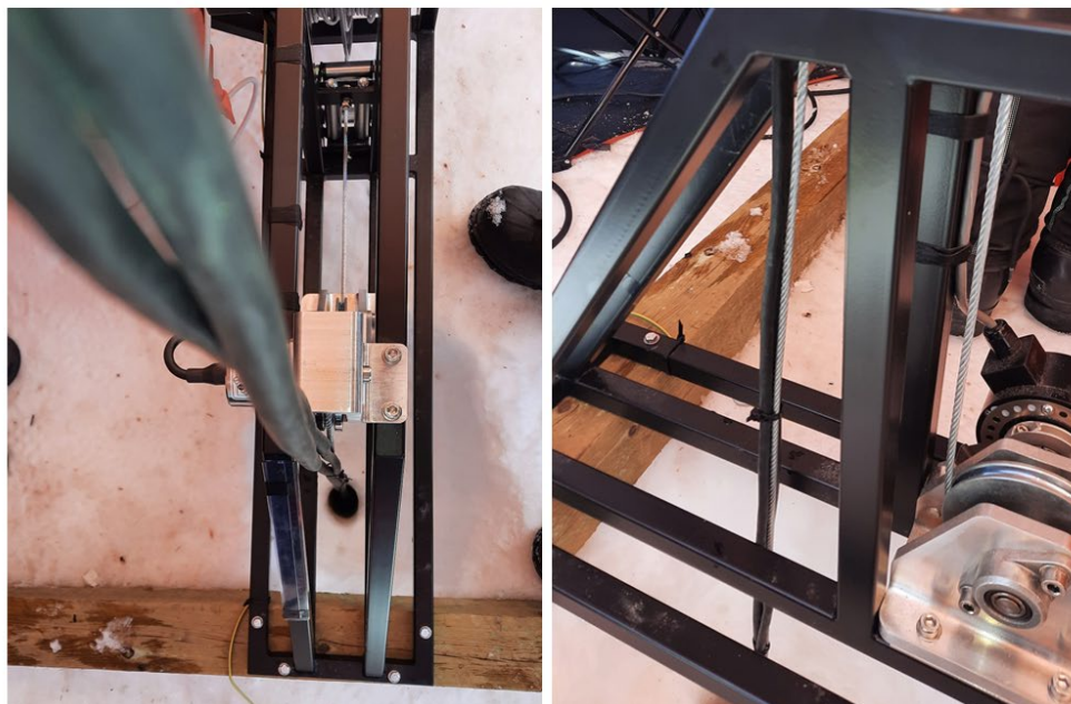
Figure 7 – Overhead (Left) and side (Right) views of the umbilical cable bundled with zip ties prior to entering the borehole.
